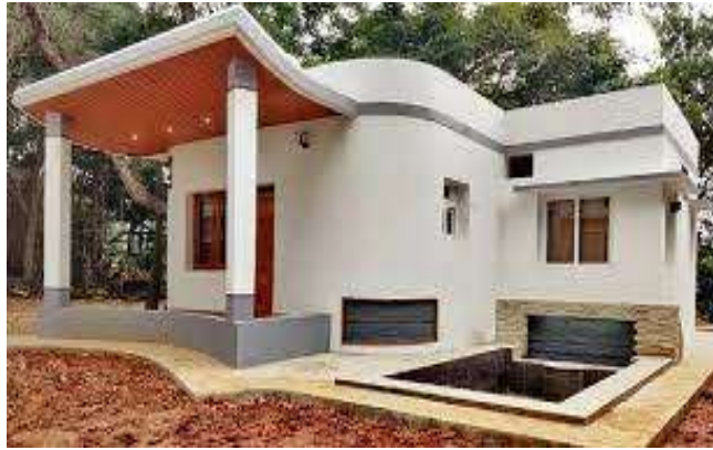
Figure 2.3 1BHK 3D concrete building by M/s Tvasta image credit Indian express .com
