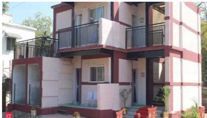
Figure 2.5 3D printed G+1 building by MiCoB image credit The Economic Times
