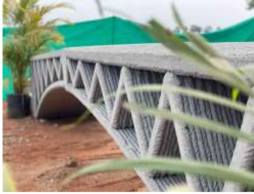
Figure 2.6 India's First Prototype 3D Printed Bridge by IIT Hyderabad. Image credit-manufactur3dmag
